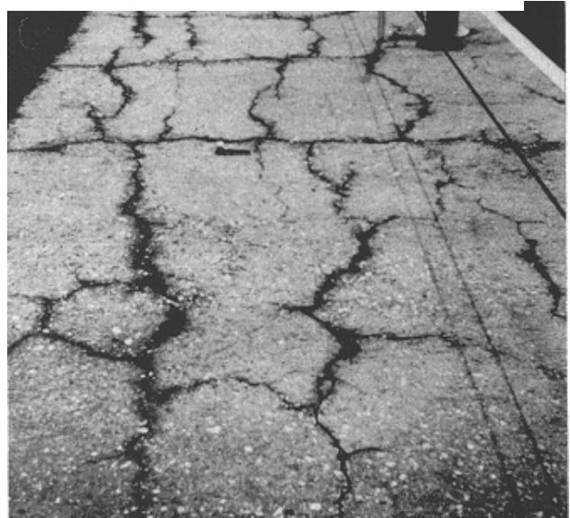
Figure 4 Pattern cracking resulting from alkali-silice reaction
