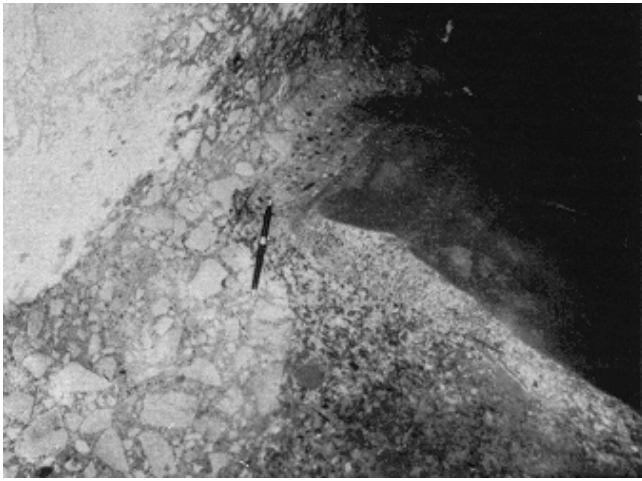
Figure 7 Smooth, worn, abraded concrete surface caused by abrasion of waterborne debris
