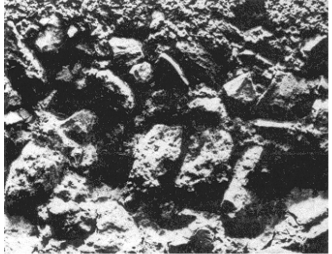
Figure 8 Rough, pitted concrete surface caused by cavitation
