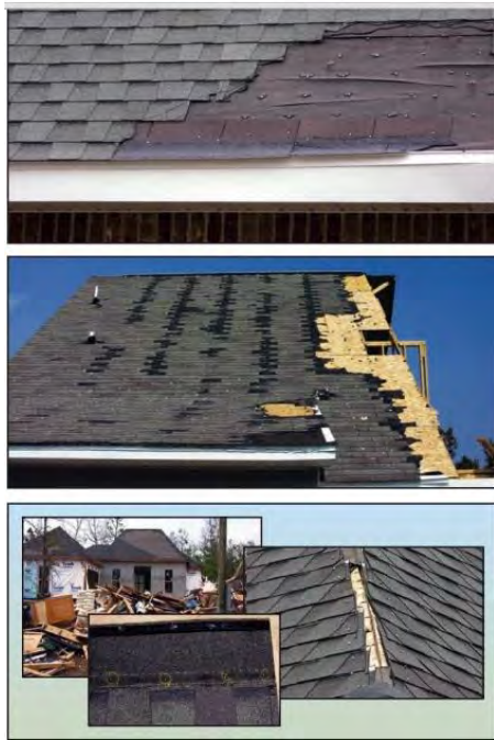
Figure 9-4: Examples of Roof Covering Loss
