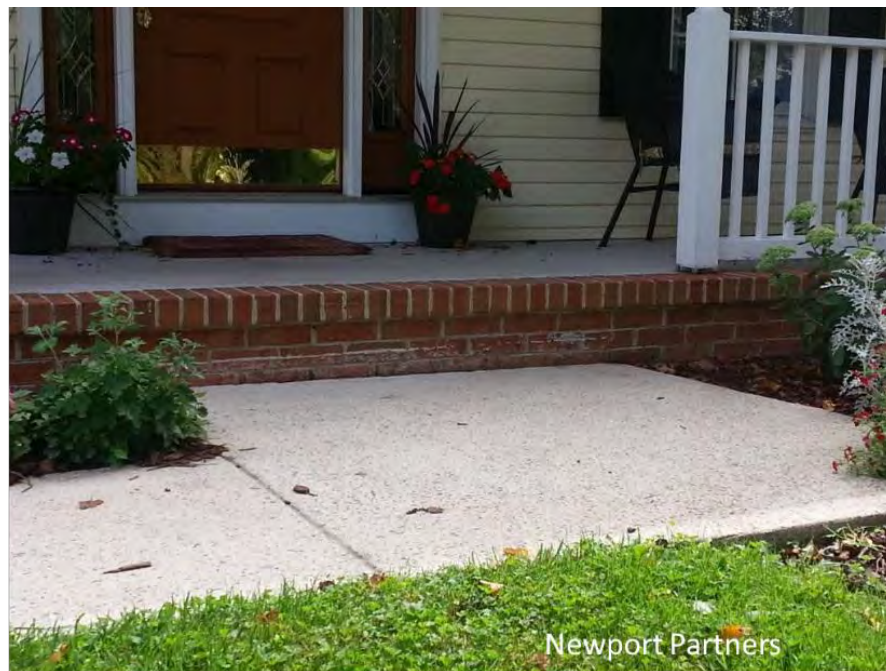
Front walkway which has settled due to insufficient compaction. Note the original concrete line against bricks, 3" higher than the current walkway elevation.
