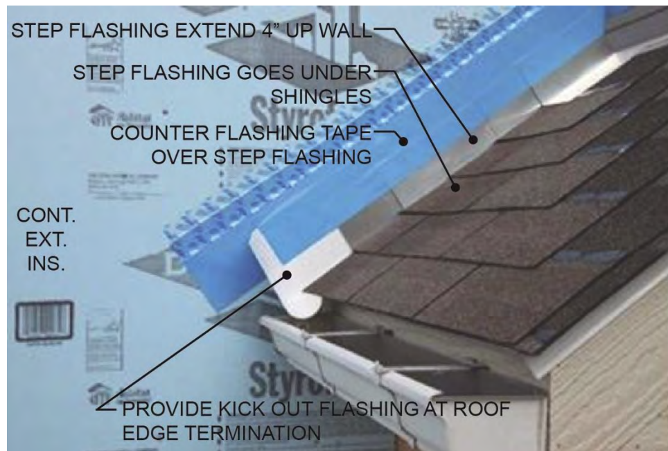
Figure 4-12: Step and Kick Out Flashing
