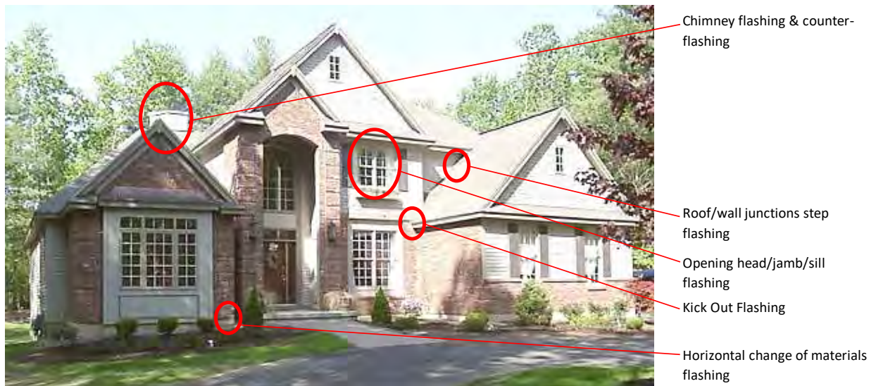
Figure 4-11: Typical Locations Where Flashing Details Are Required
