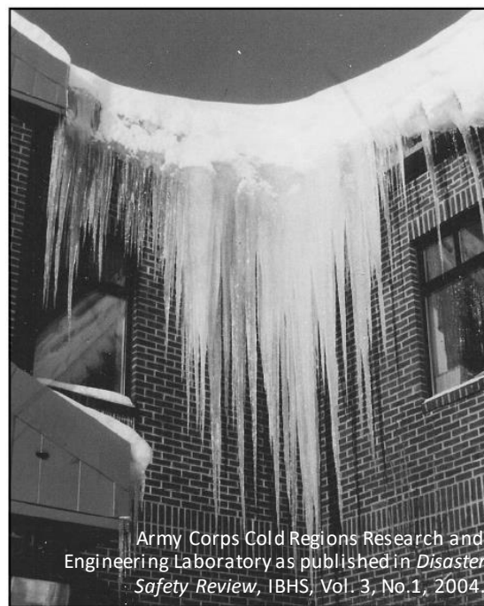
Figure 4–6: Example of a Severe Eave Ice Dam
