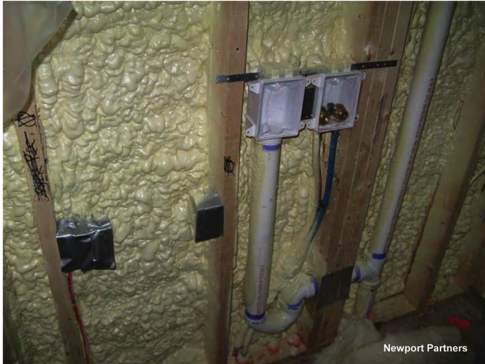
Example of plumbing lines well protected from freezing because of high R-value, low air-infiltration spray foam insulation between the pipes and outdoors.
