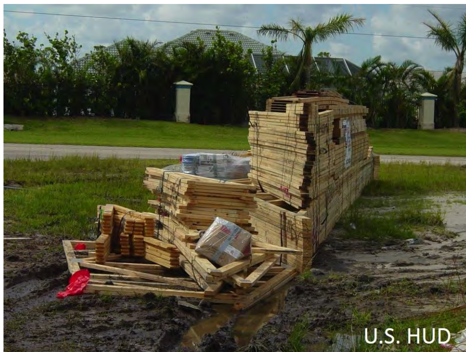
Figure 4–21: Example of Unacceptable Construction Material Storage
