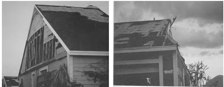
Figure 9–1: Examples of Roof and Building Damage From High Winds
