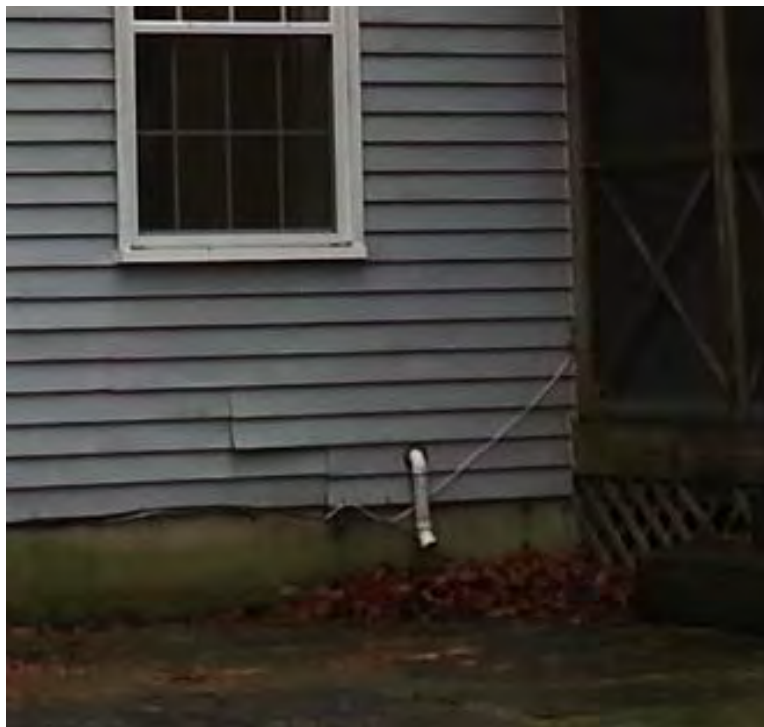
Figure 9–7: Sump Pump Discharge Right Next to Foundation
