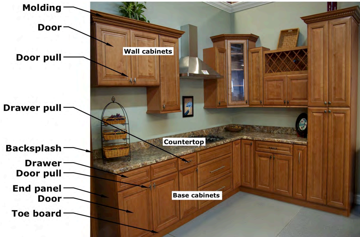
Figure 2.22 Components of typical kitchen cabinets
