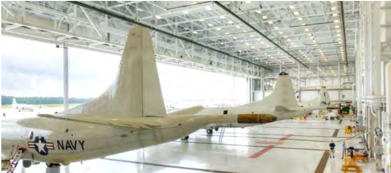
Figure 3.31 Jacksonville Naval Air Station P302V Maintenance Hangar. To meet the US Navy's demand for multiple openings for various aircraft, clear spans of 455 feet and 428 feet were necessary at the front of the hangar. To achieve these record-setting clear spans, heavy structures utilized three-story tall box trusses to design the hangar. During erection, these robust trusses were assembled in sections on the ground then lifted into place with the entire system bearing on temporary shoring towers. The structure also supports multiple overhead cranes for maintenance of the aircraft. The 3-D structural design by Heavy Structures proved to be over 25% more efficient than the nearest conventional solution. The size, complexity and economy of this successful project demonstrates the capabilities and advantages Heavy Structures has to offer. (Source: Butler Manufacturing)
