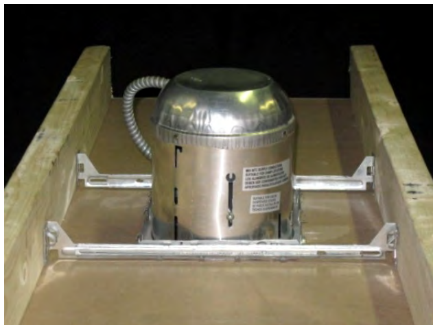
Figure 1.9 A properly installed IC-rated recessed or 'can' light which can be safely covered with insulation.
