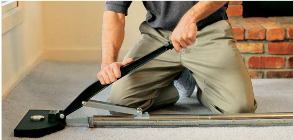
Figure 2.13 stretch-in installation
