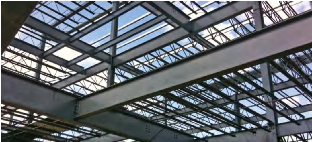
Figure 3.28 A conventional metal structure is ready to be completed with metal systems encompassing all conventional steel products — ranging from wide-flange beams and bar joists to pipes and tubes. This production is a good example of the kit-of-parts approach where all parts are standardized. (Source: Butler Manufacturing)
