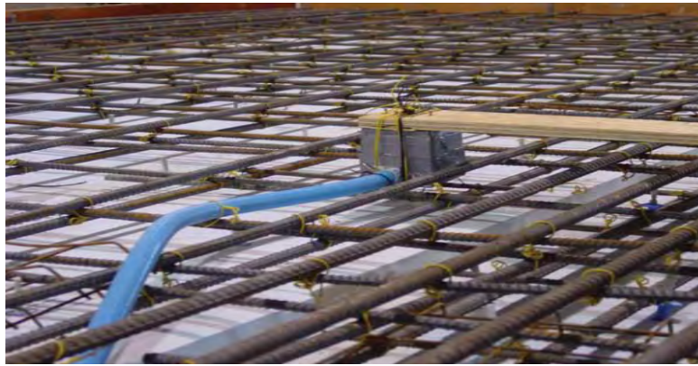
Figure 3.34 Electrical conduit and outlet box being installed in insulated sandwich wall pane
