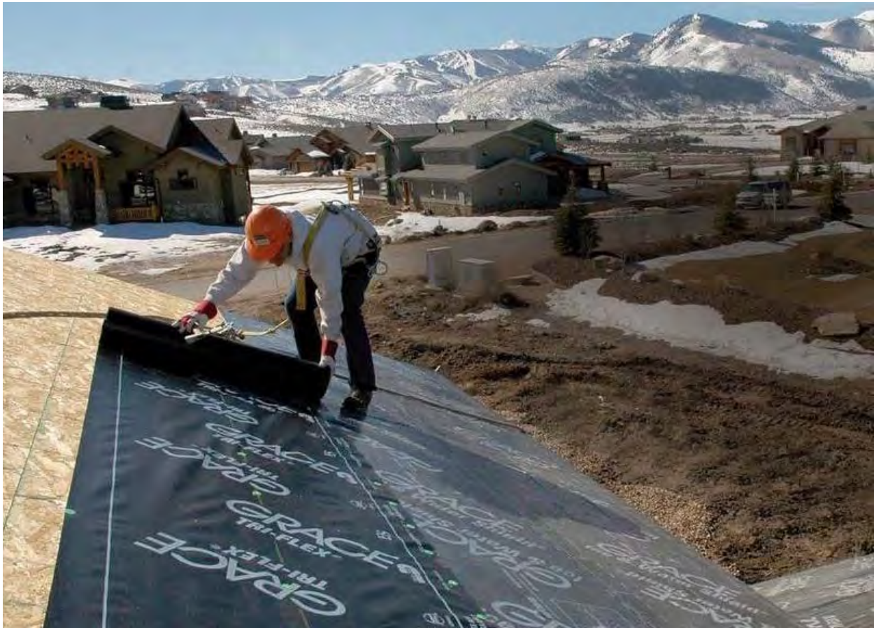
Figure 2.3 Asphalt felt roll installation
