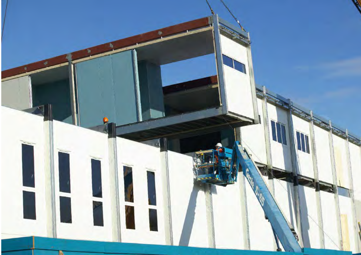
Figure 3.18 Technically advanced modular steel installation: The modules can be stacked vertically and horizontally on one another. The floor area can be therefore reduced or increased based on the required program. (Source:
