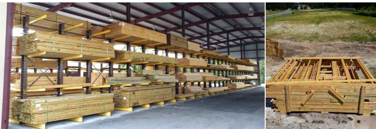
Figure 3.6 Left: Covered inventory. Right: Panelized wood walls before installation. (Source: Panel Tek)
