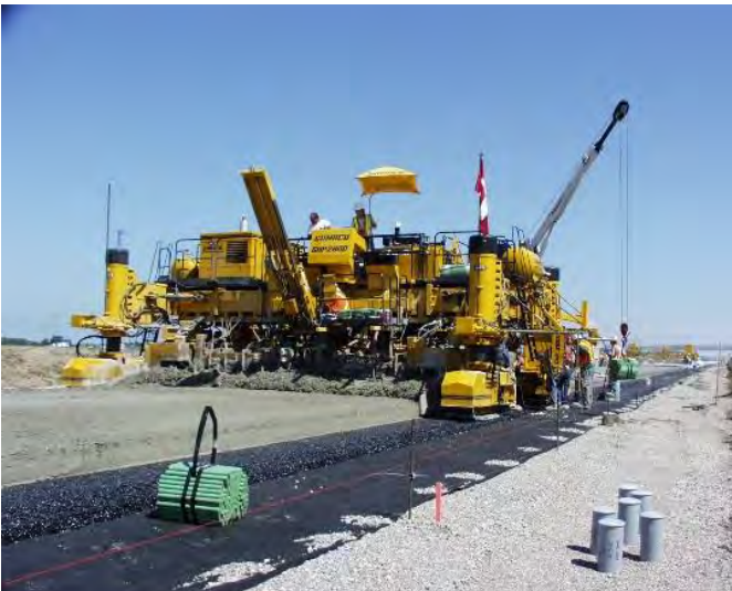
Figure 8. Photo. Base extended beyond the concrete pavement to provide support for the paving equipment.
