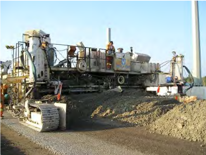
Figure 7. Photo. Cement-treated open-grade drainage layer.
