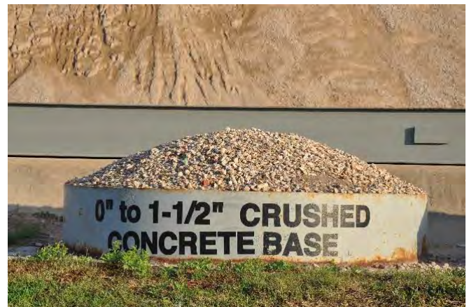
Figure 9. Photo. Reclaimed concrete crushed to be used as a base for concrete pavements.
