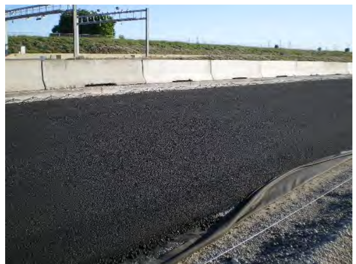
Figure 6. Photo. Asphalt-treated base.
