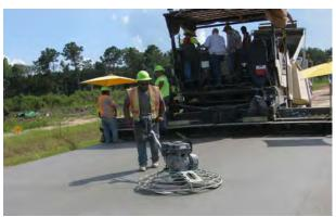
Figure 12. Method to improve upon RCC finished surface.
