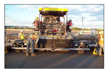
Figure 8. High-density RCC paver.
