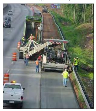
Figure 9. RCC construction.
