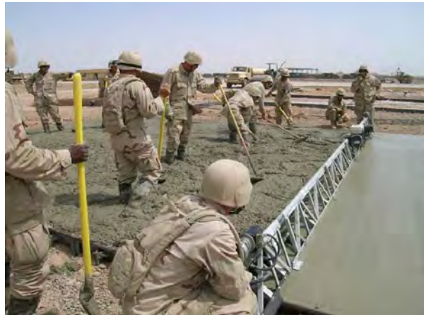
Figure 66 – Mechanical screed.
