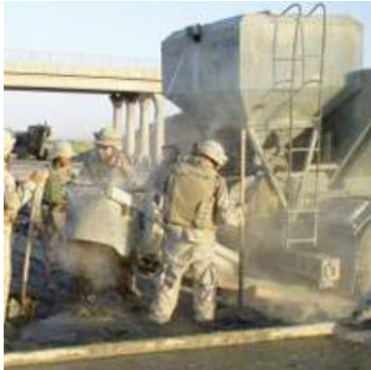
Figure 11 – Aggregate batching plant.
