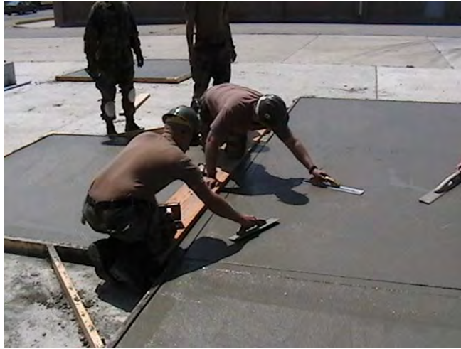
Figure 70 – Hand float in use.
