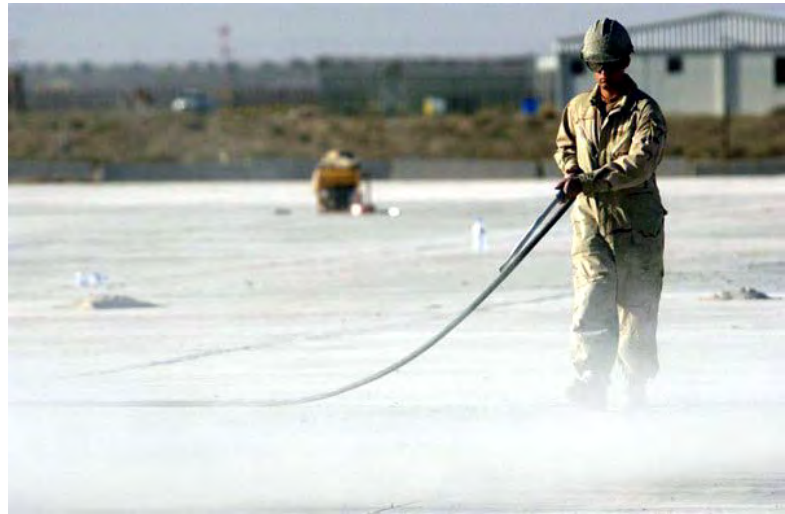
Figure 78 – Sprinkling concrete with water.
