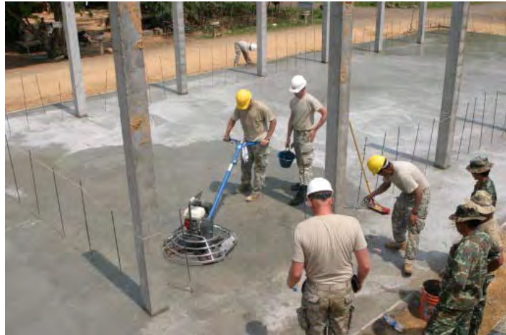
Figure 76 – Mechanical troweling machine.
