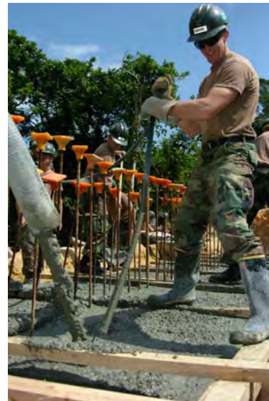
Figure 63 – Using a vibrator to consolidate concrete.
