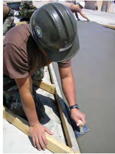
Figure 73 – Edger in use.
