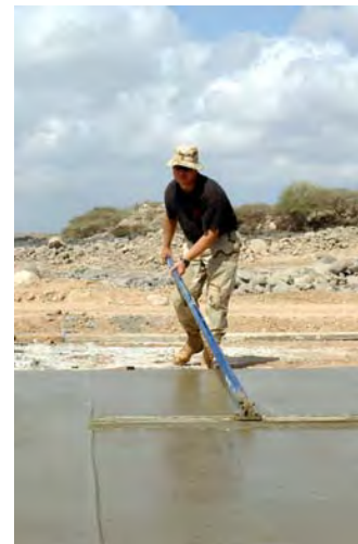
Figure 71 – Long handled float in use.
