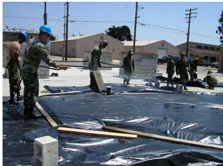
Figure 79 – Curing concrete with plastic.
