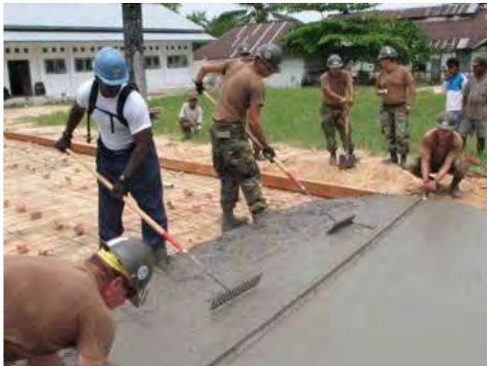
Figure 65 – Screeding operation.
