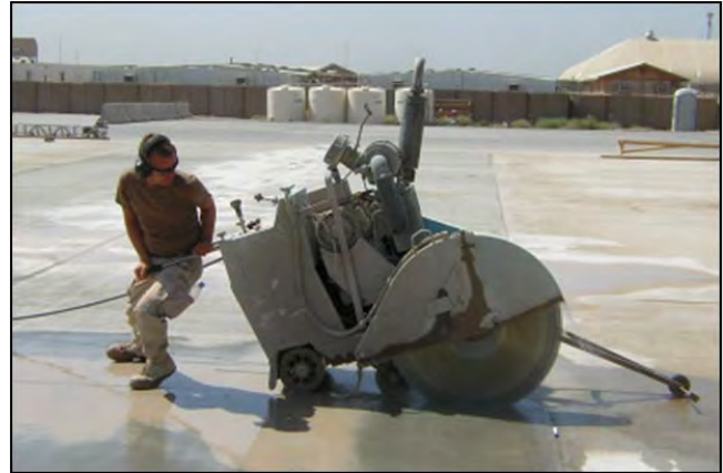
Figure 61 – Concrete saw.
