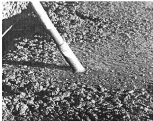
Figure 64 – Consolidation by an internal vibrator and a spading tool.
