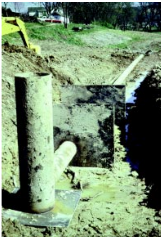
Figure 22 Drop-inlet pipe spillway with antiseep collar
