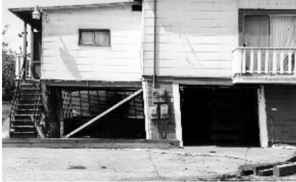
Figure 2-15 House experiencing soft- and weak-story behavior in the Cape Mendocino earthquake. Deformed shape of garage door opening shows approximately 6 inches of horizontal movement in the first story.
