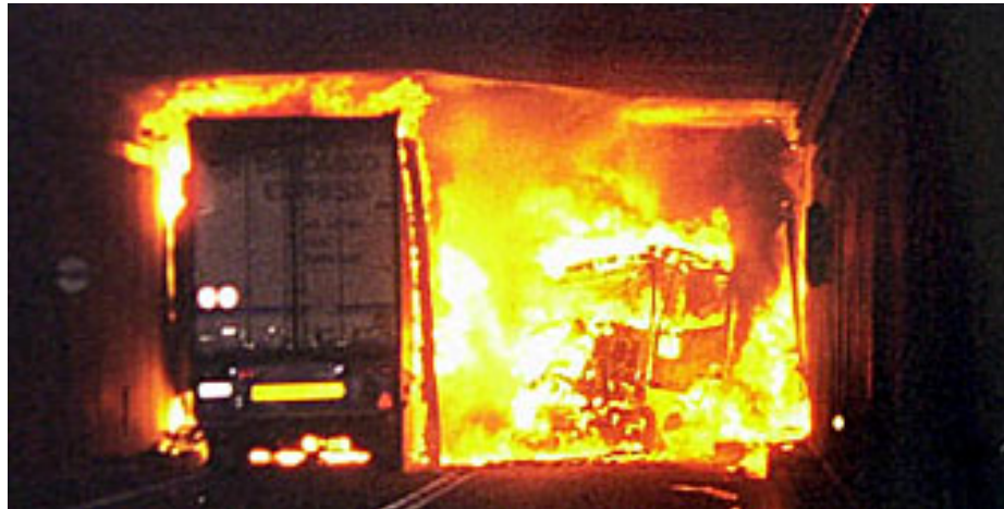
Figure 1-11 Gotthard Tunnel Fire in October 2001 (FHWA 2006)
