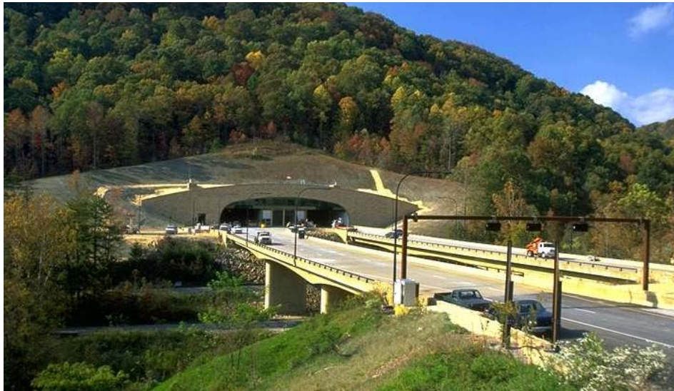
Figure 2-8 Portal Structure for Cumberland Gap Tunnel
