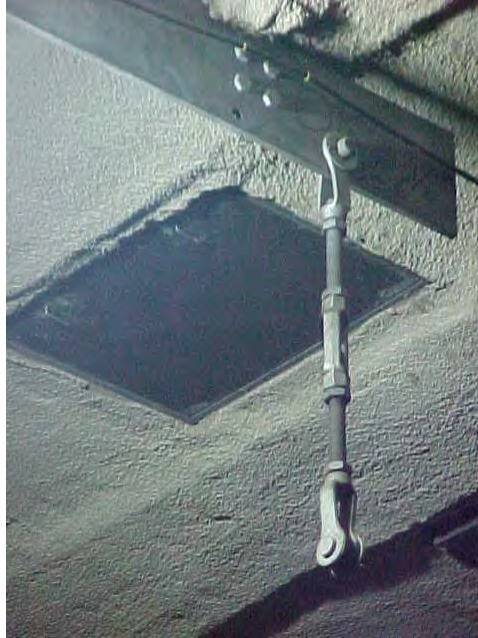
Figure 16-22 Typical Replacement Hanger Hardware
