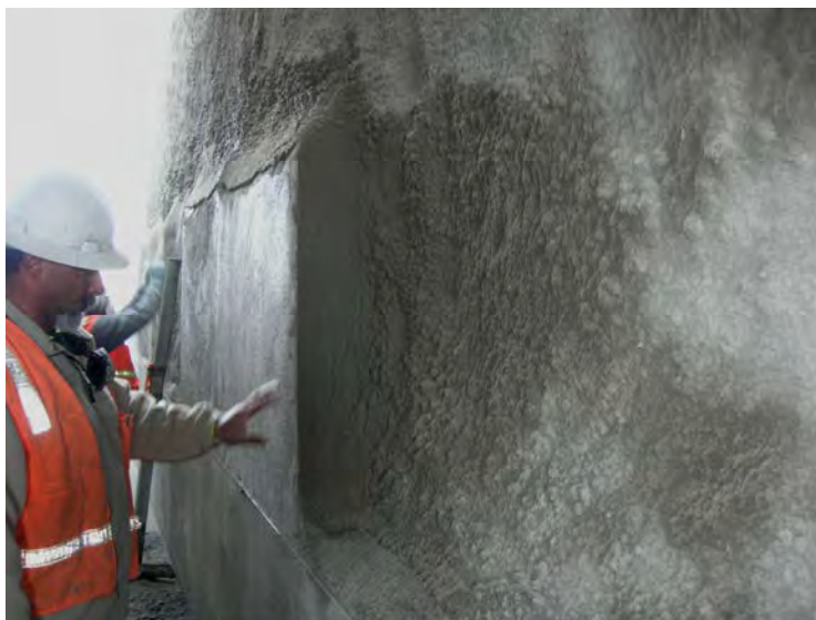
Figure 16-13 Shotcrete Finishing, Shawmut Jct. Boston
