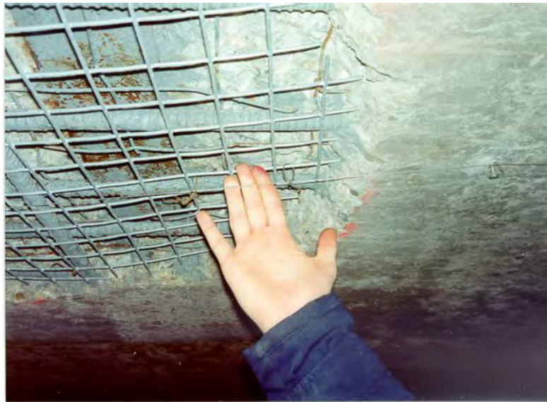
Figure 16-12 Reinforcing Steel for Repair, Sumner Tunnel Boston
