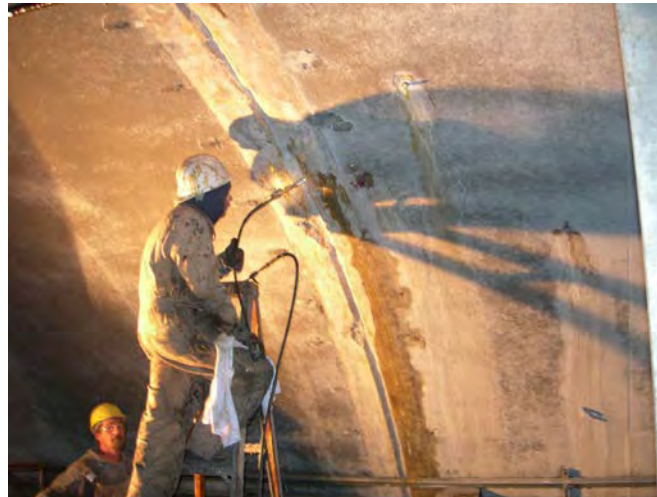
Figure 16-4 Leak Injection, Tuscarora Tunnel PA Turnpike
