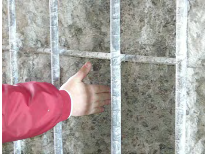
Figure 16-7 Substrate after Hydro-demolition, Shawmut Jct. Boston
