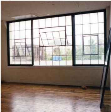
Fig. 15. Original steel windows were retained and made operable during the rehabilitation of this historic mill complex. Insulated sliding windows were added on the interior to improve energy efficiency.
