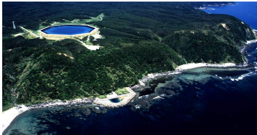
Figure 13. J-Power's ocean PSH in Okinawa, Japan. 31
