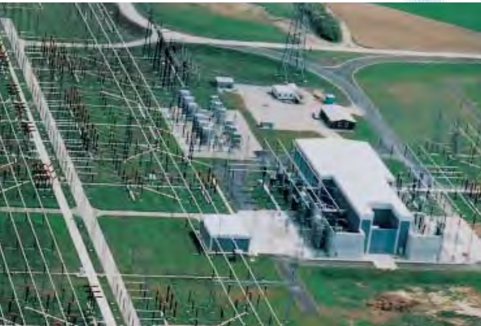
Fig. 2-3: Back-to-back converter Station Vienna Southeast
