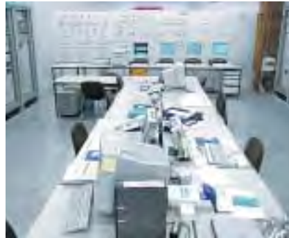
Fig. 5.7.1-11: Example for a functional performance test setup
