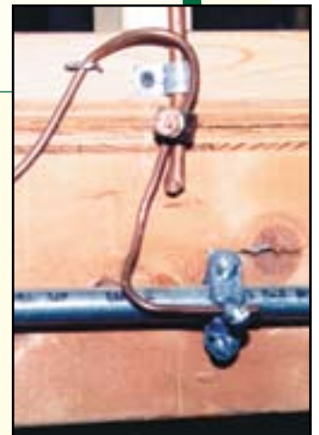
Install bonding jumpers around nonconductive material.
