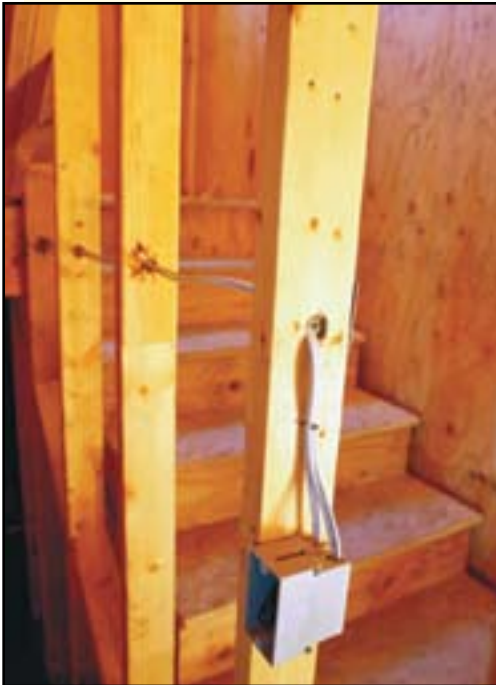
Nonmetallic sheathing helps protect wires from damage.
