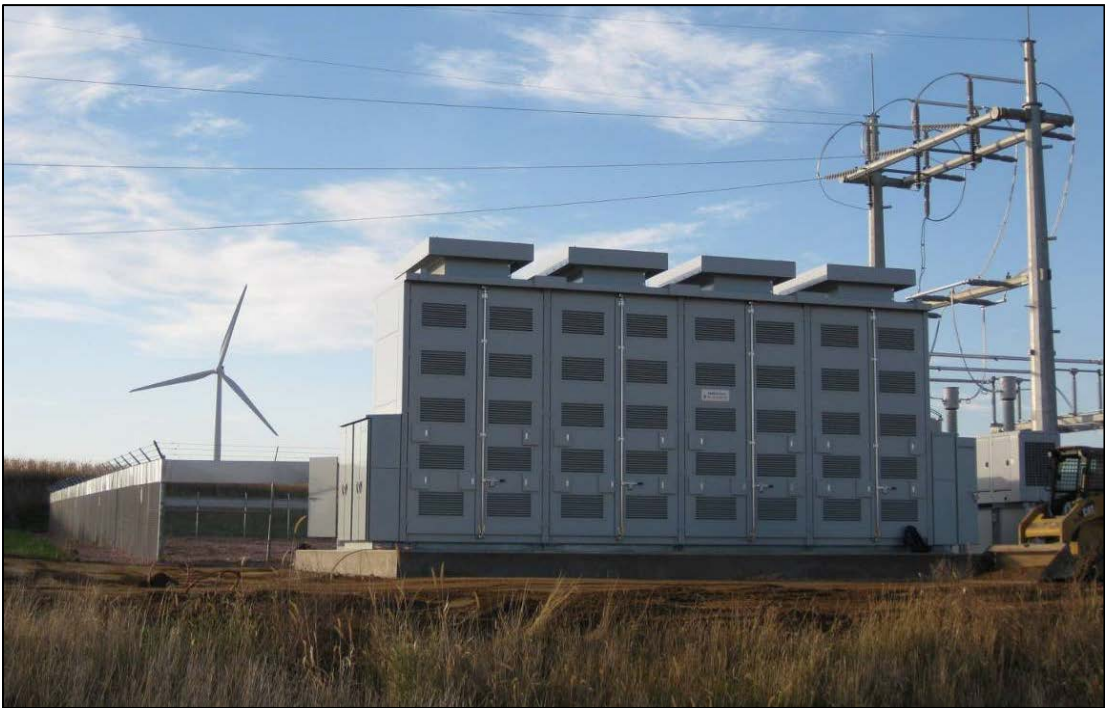
Figure 34. Xcel Battery Supplementing Wind Turbines, Lucerne, MN
