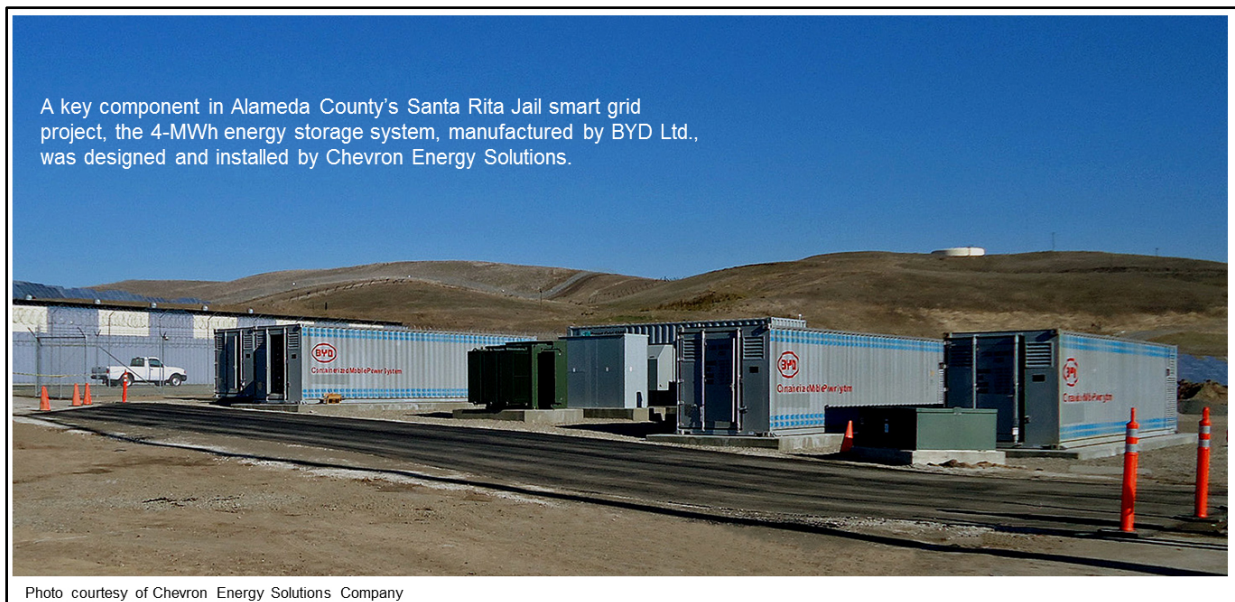
Figure 98. A 2-MW/4-MWh Li-ion Energy Storage System
