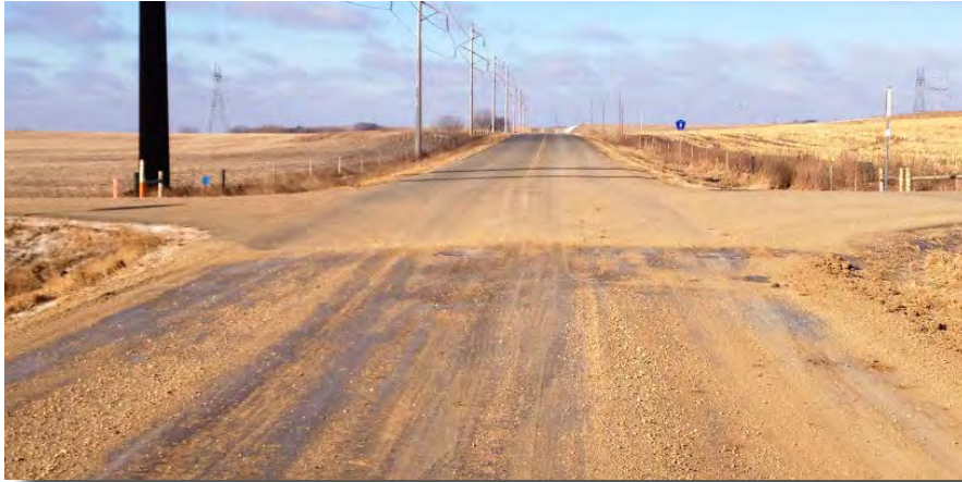
Another area prone to develop washboard or potholes is a transition from gravel to paved surface.
