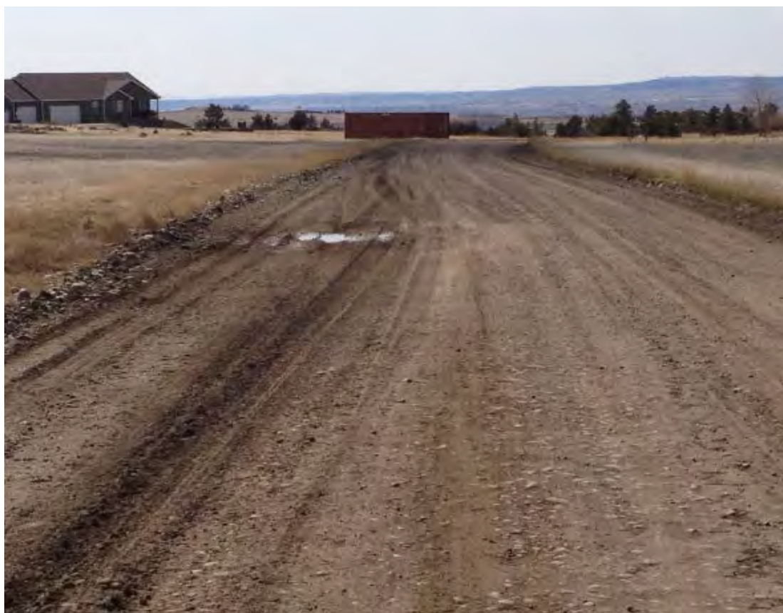
This road has a poor cross section. Drainage is important, even though the road is located in a semi-arid region.
