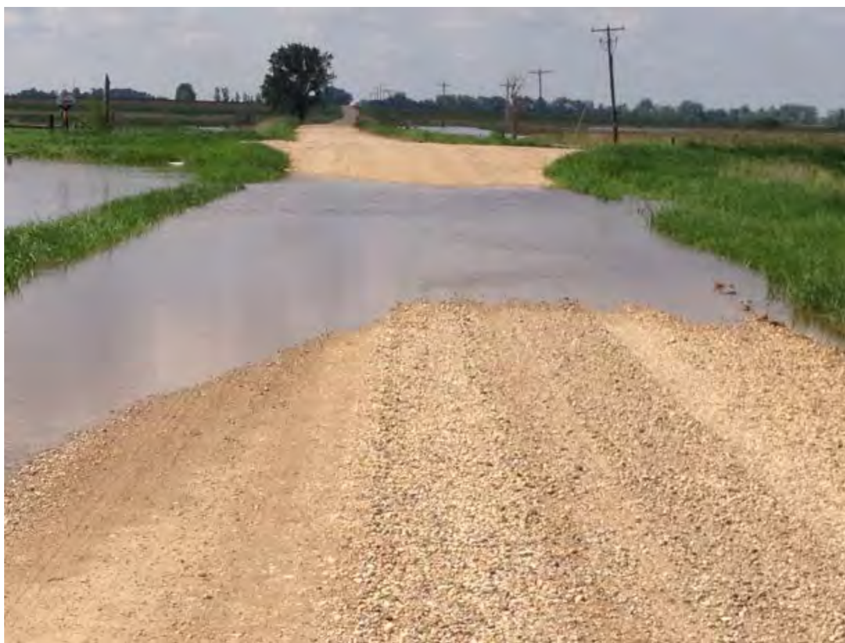
Plugged or collapsed culverts cause serious damage when water flows over roads.
