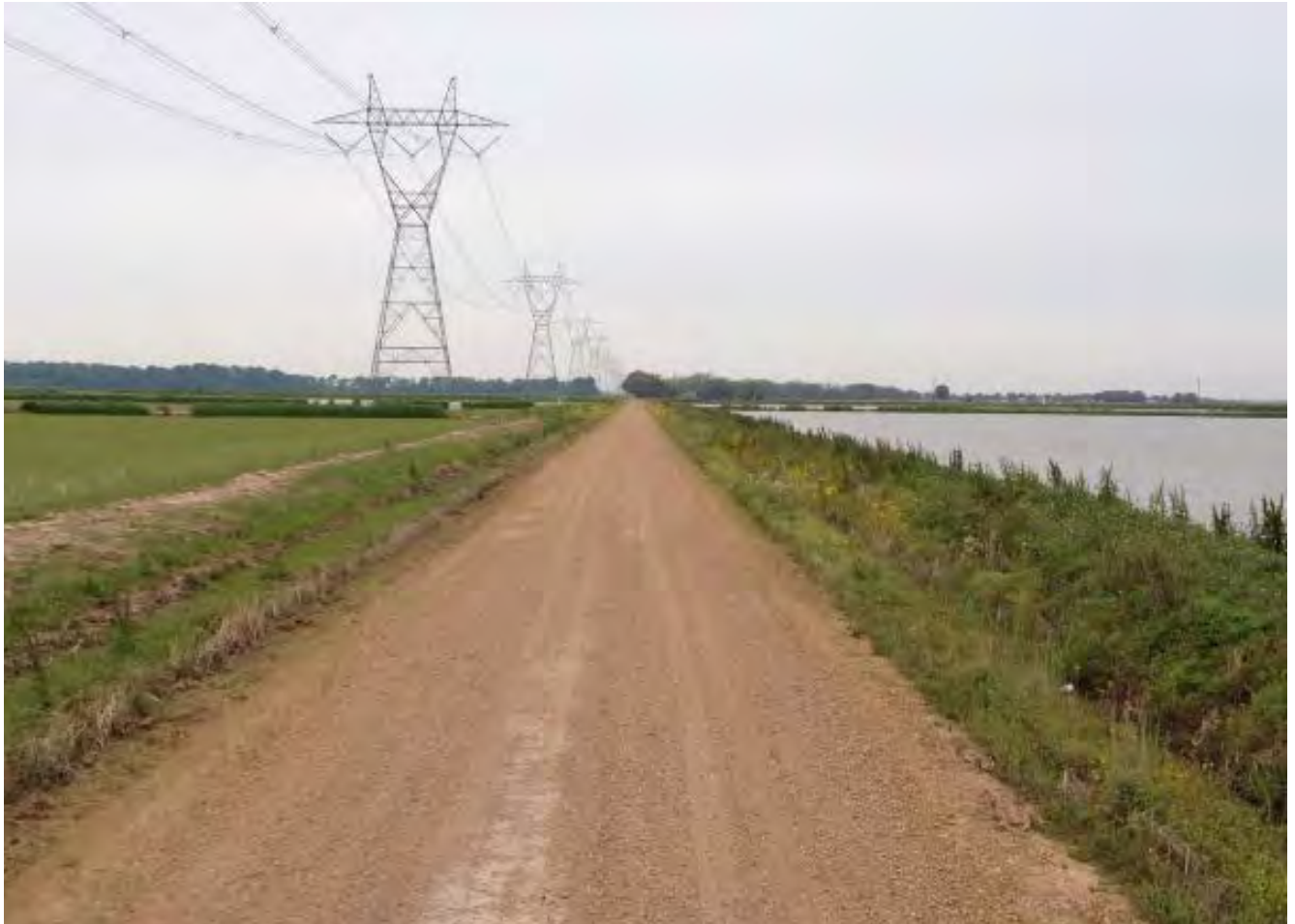
This road performs remarkably well because of good crown and good gravel quality in a very wet region.
