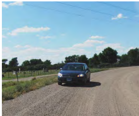
Well-shaped superelevation on a curve.
