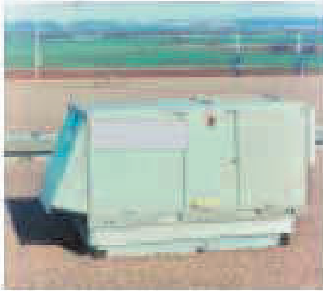
Figure 11: Small rooftop air handling unit.
