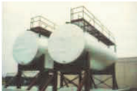
Figure 59: Horizontal tanks including concrete-lined tanks.
