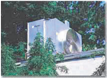
Figure 35: Fluid cooler cross flow with self-contained sump.
