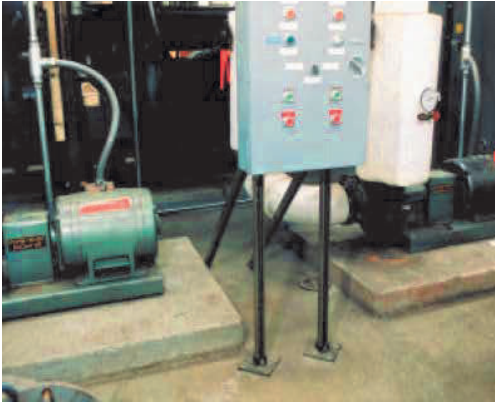
Figure 155: Typical control panel support using angles. Additional angle supports may be required (see below).
