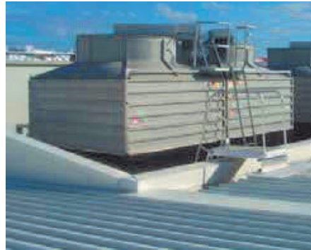
Figure 36: Cooling tower with self-contained sump.
