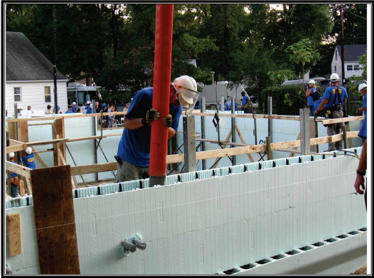
House Construction Using Insulating Concrete Forms
