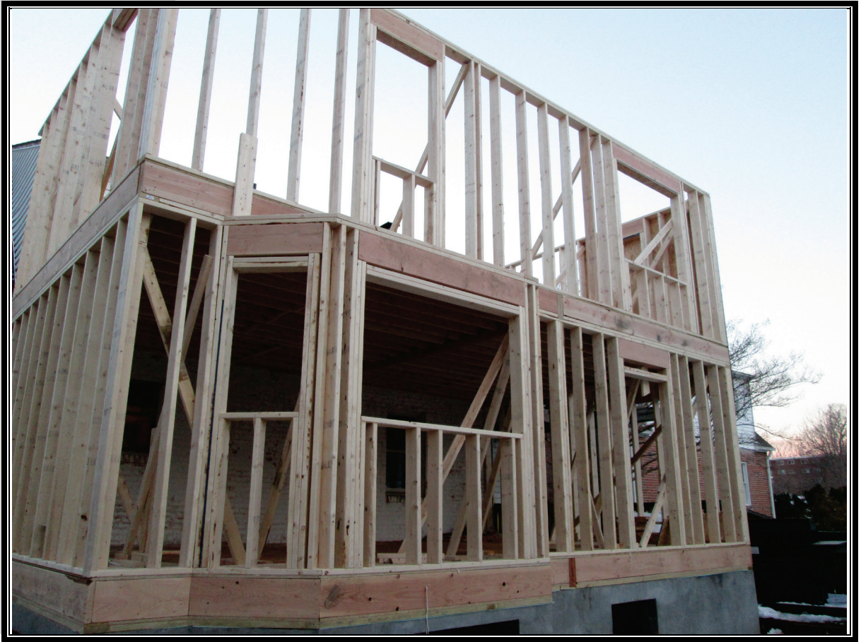
FIGURE 1.2 Modern Platform-Framed House Under Construction
