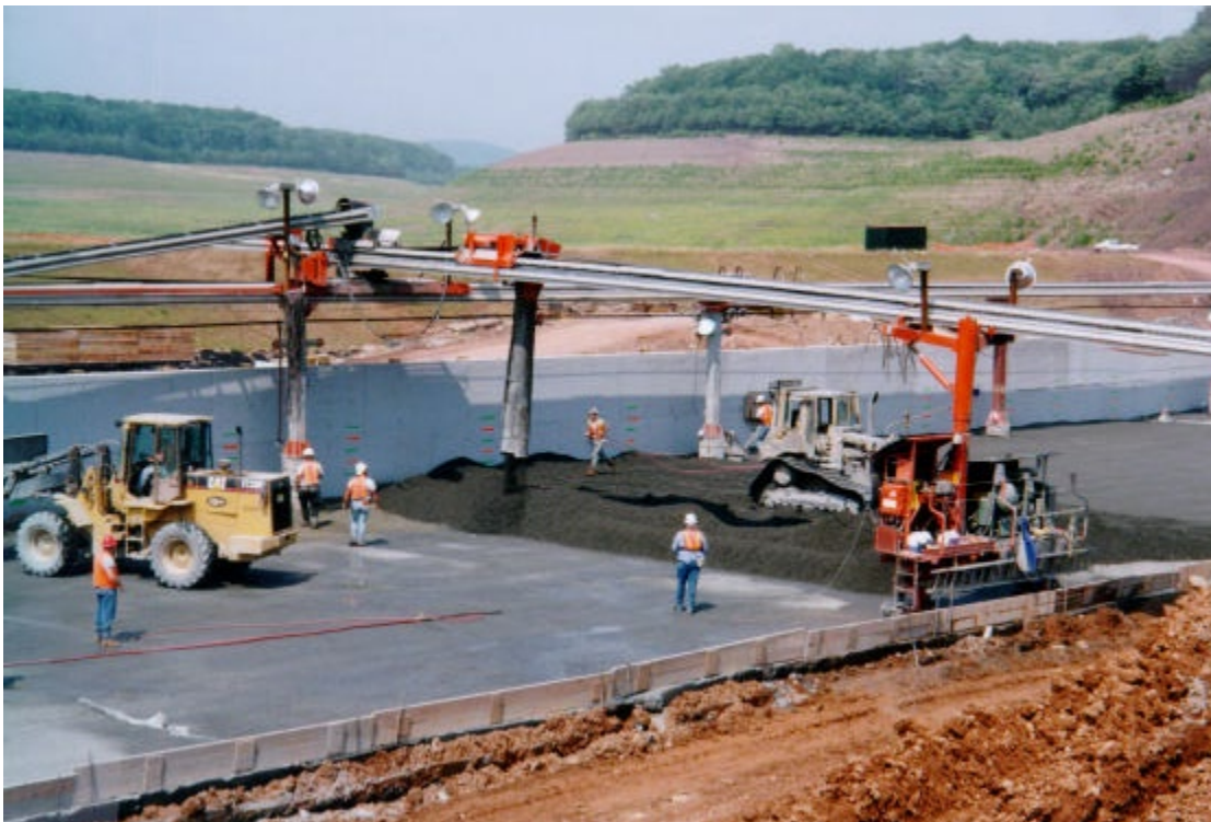
Figure 6-2. Conveyor system with mobile side discharge belt
