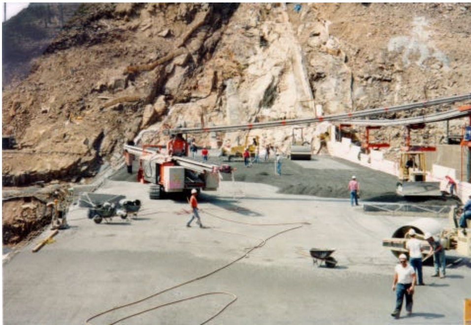
Figure 6-1. Conveyor system with self-propelled crawler-placer
