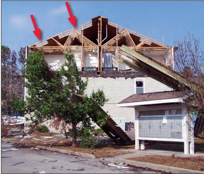
Figure 2-12. Failure of the gable end wall of this apartment building led to pressurization of the attic and the release of sheets of plywood sheathing. Note the plywood roof sheathing “unzipped” by wind pressures (arrows), (Ocean Springs, Mississippi).
