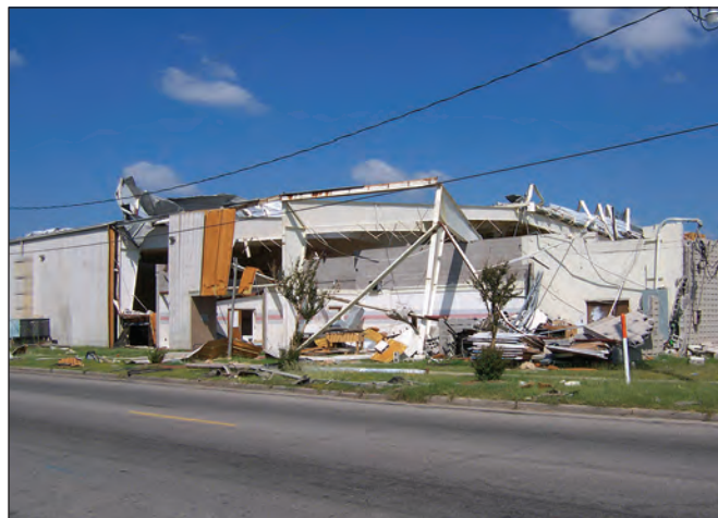
Figure 2-16. Pre-engineered metal building failure (Gulfport, Mississippi)
