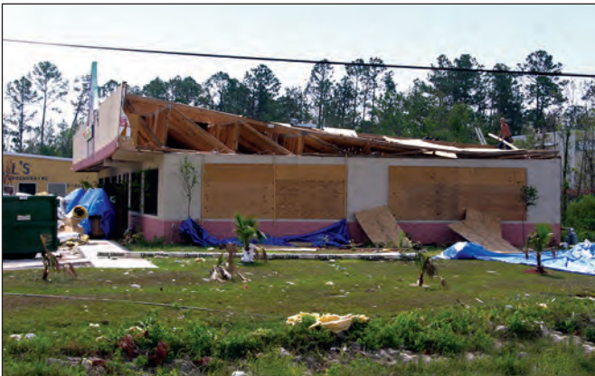
Figure 2-13. Failure in a wood frame commercial building. Trusses lost roof sheathing, allowing trusses to tip over (Ocean Springs, Mississippi).
