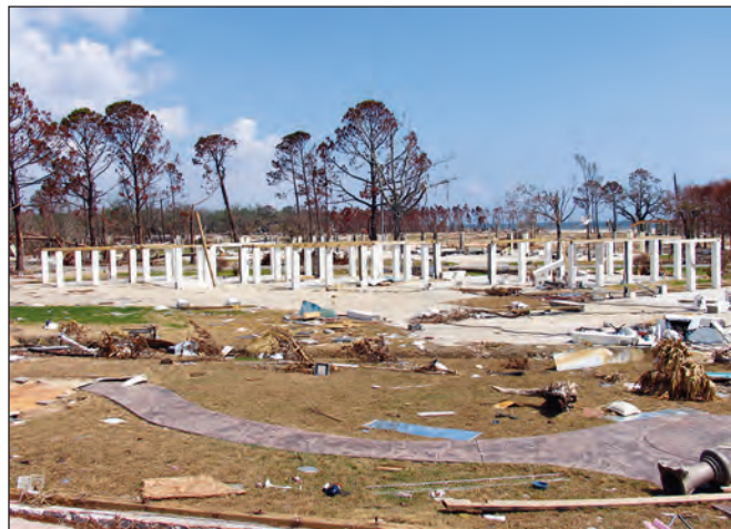
Figure 2-3. Typical building failures when surge and waves exceeded pier foundation height (Long Beach, Mississippi)
