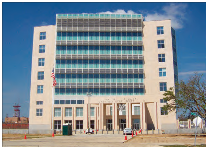
Figure 2-15. Reinforced concrete/steel frame building that performed well structurally, but did have some building envelope damage and roof mounted HVAC equipment damage (Gulfport, Mississippi)
