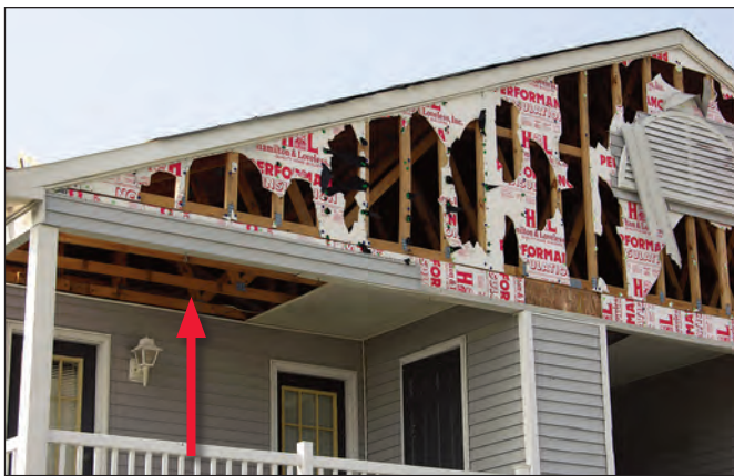
Figure 2-19. Loss of vinyl siding and foam insulation at a gable end wall. Note the missing vinyl soffit (red arrow). Not visible was the loss of roof sheathing caused by progressive failure that was initiated by soffit loss (Long Beach, Mississippi).
