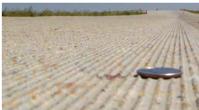
Figure 5.11 Diamond-ground texture (Rasmussen et al. 2008)
