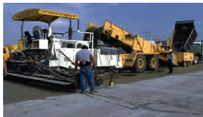
Figure 5.14 RCC placement (Harrington et al. 2010)
