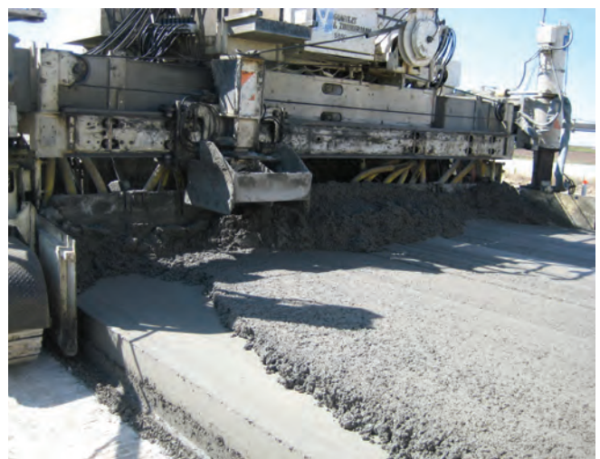
Figure 3.2 Two-lift pavement being constructed in Kansas
