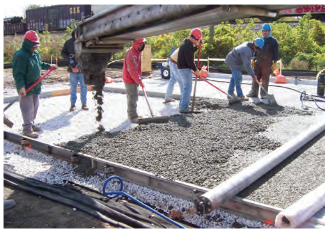
Figure 3.7 Pervious concrete being placed (photo courtesy of John Kevern, University of Missouri-Kansas City)
